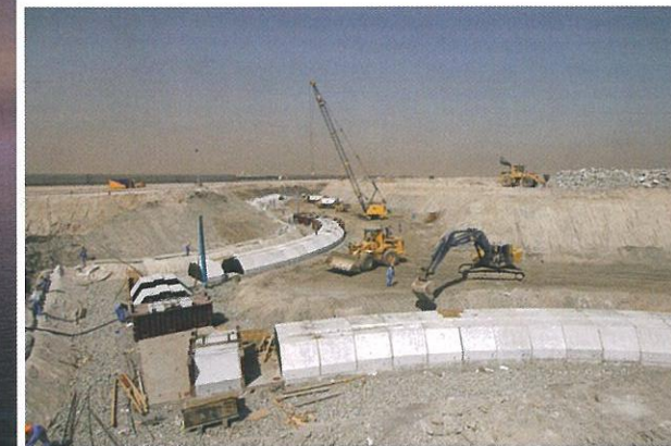
Infrastructure work has commenced Below: Farhan Faraidooni
